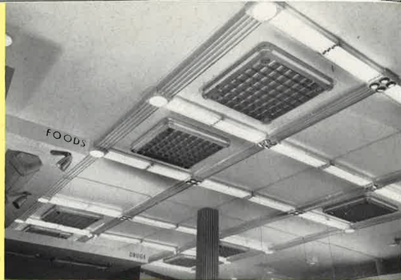
CONTINUOUS LINES CROSSWISE. Standard line 40-watt T-12 fluorescent and 6-foot T-8 Slimline lamps of same brightness may be switched on, to compare the crosswise shielded view with the endwise view of lamps as illustrated in photo at left.
