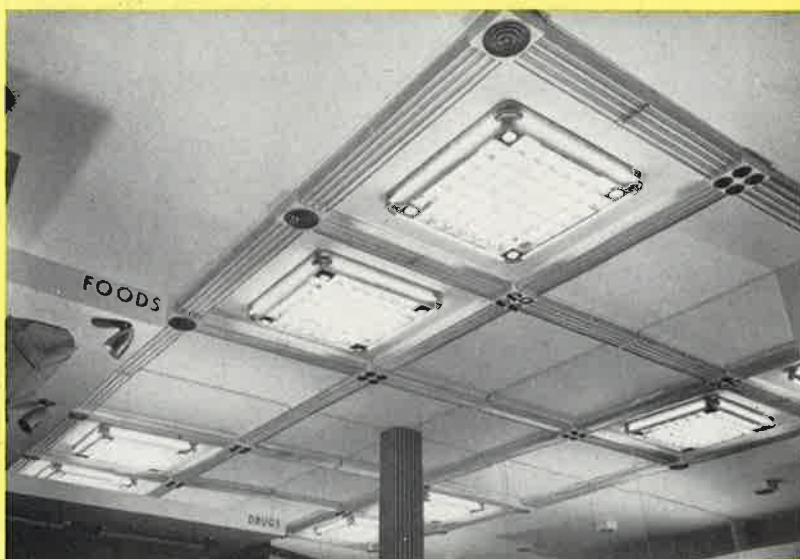
SYSTEM OF DIFFERENT CHARACTER may be appraised with square units. Inner elements have 35^\circ shielding in both directions. Projector spots in gimbals. Exposed low-brightness 40-watt T-17 fluorescents on sides reduce contrast of luminaire with ceiling.
