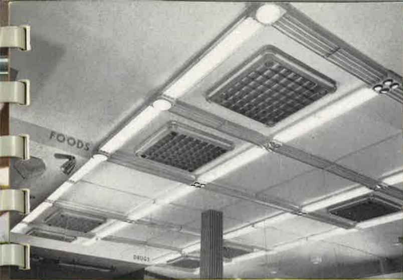
CONTINUOUS LINES LENGTHWISE. Slimline fluorescent lamps of 8-foot and 6-foot length operated at 200 ma. with filament downlighting integrally interspersed. Crosswise shielding of 35^\circ . All fluorescent lamps used are 4500^\circ white.
