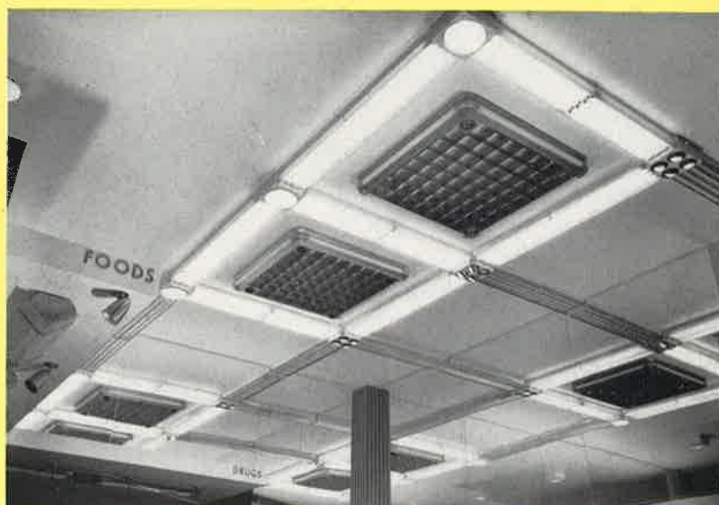
SIXTY FOOTCANDLES of fluorescent light supplied by this pattern. Groups of louvered projector spots in gimbals provide two or more times that amount for selling or display areas. Gimbals permit aiming the beam in any direction within 30^\circ from vertical.
