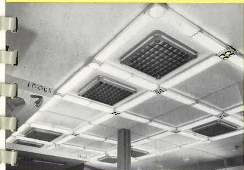
COMPLETELY CONNECTED PATTERN obtained by adding the 6-foot Slimline luminaires demonstrating illumination of 100 footcandles. The downlighting may be turned on and off to observe its contribution to quality and appearance of merchandise.
