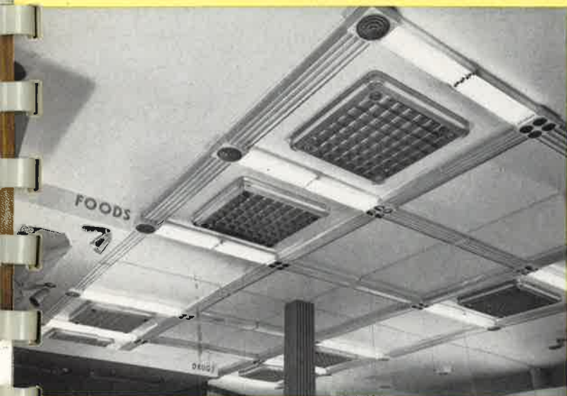
INTERRUPTED PATTERN of two luminaires for 40-watt fluorescent lamps in tandem. These provide a basic level of 30 footcandles. Large downlights have 500-watt filament lamps in mirrored-glass reflectors with glass covers and concentric louvers.
