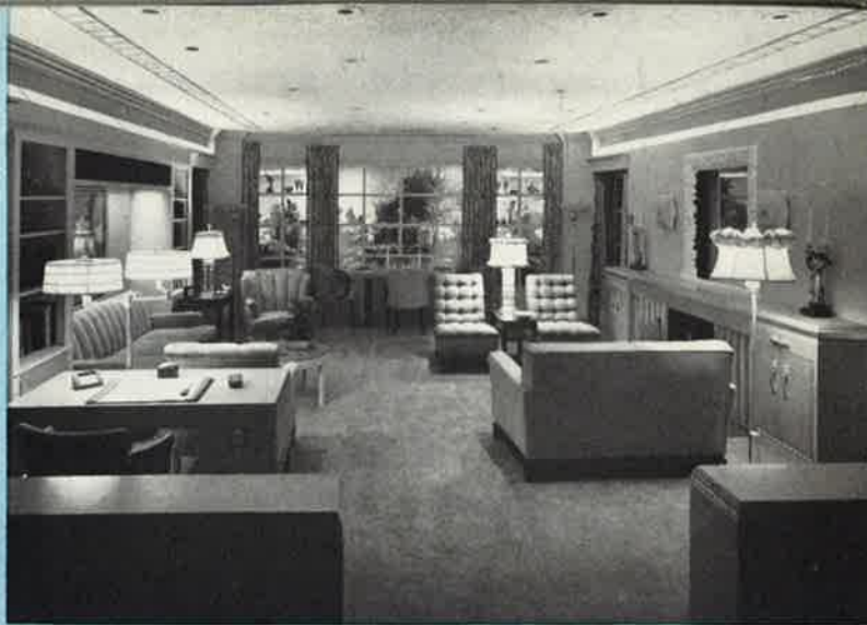
A FAMILY'S BUSY EVENING at home needs functional lighting to suit the deed (30 to 125 ft-c from lamps and seven downlights), held in comfortable balance by the cove lighting. 2,200 watts in use.
