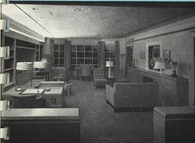
ONE COVE is demonstrated to show its unusual light distribution across ceiling and opposite wall which when balanced (opposite) results in previously unrealized smoothness and effectiveness. Uses 204 watts.
